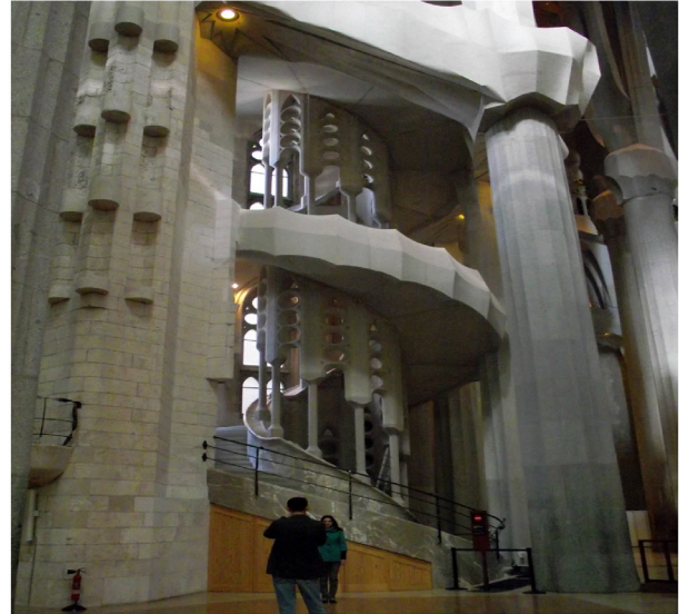
Fig. 5 - Helicoid, (Diagram on the left in http://en.wikipedia.org/wiki/ Helicoid ) applied in stairs, Sagrada Família, Barcelona.
