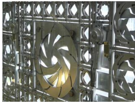
Fig.10 – Pormenor do sistema da janela – Fonte: http://www.archdaily.com/162101/ad-classics-institut-du-monde-arabe-jean-nouvel/4125486394_56b2a2bb04_oboonj/
