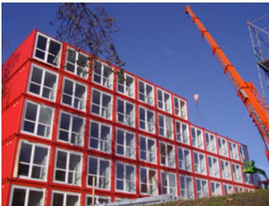
Figure 6 - Keetwonen in construction, Amsterdam
