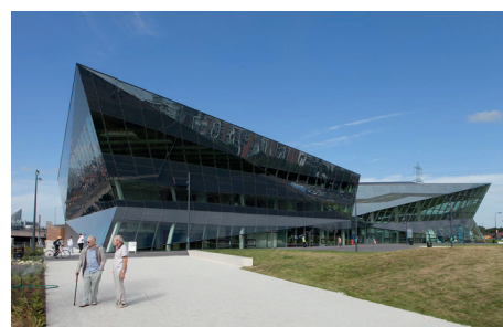
95. Fachada do edifício The Crystal, Wilkinson Eyre Architects.
