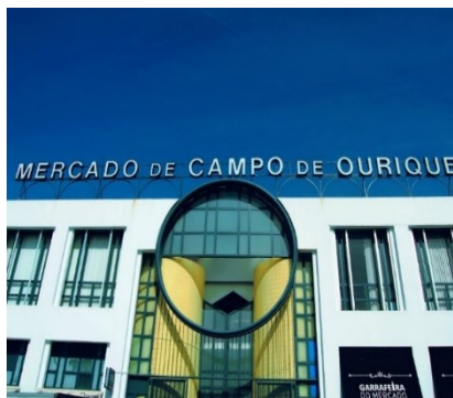
Fig. 7- Southern entrance of the Campo de Ourique Market
