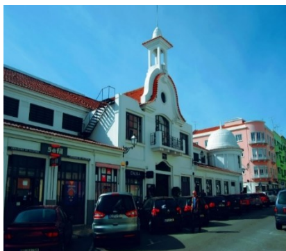
Fig. 6- Eastern façade of the Campo de Ourique Market
