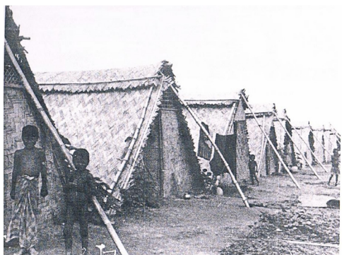
Fig. 11. A-Frame Construction, Demra, Bangla Desh (Davis, 1980, p. 91)
