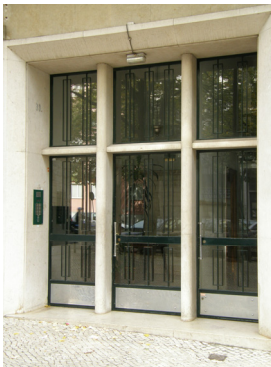
Door of building
