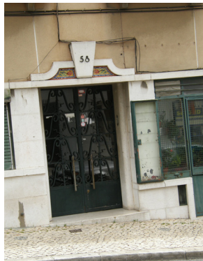
Door of the building
