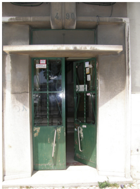
Door of the building
