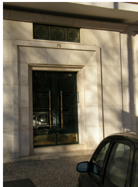
Door of the building
