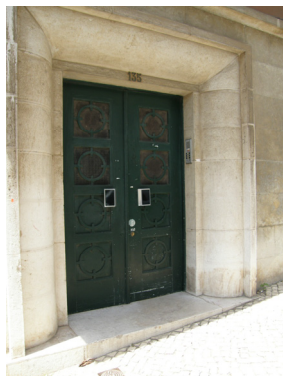
Door of the building
