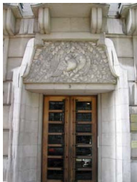
Door of the building
