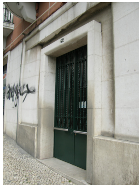
Door of the building
