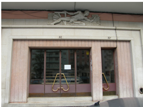
Door of building
