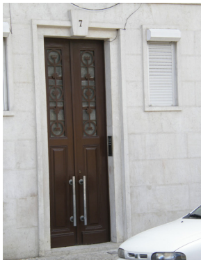
Door of the building
