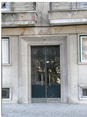
Door of building
