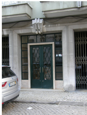
Door of the building
