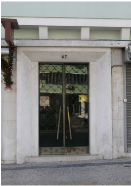
Door of building
