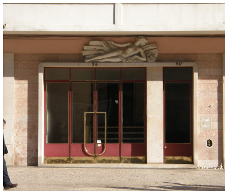
Door of building
