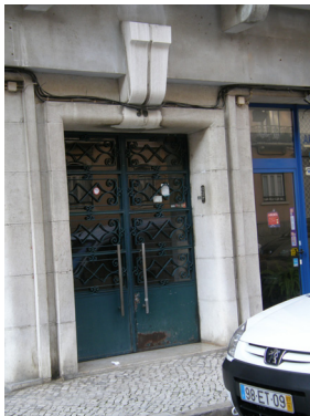
Door of the building
