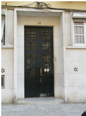
Door of the building
