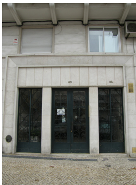
Door of building
