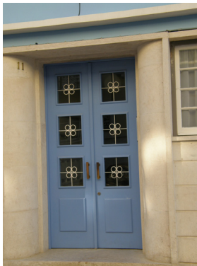
Door of the building
