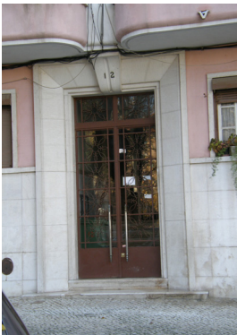
Door of building
