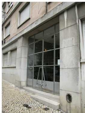
Door of the building
