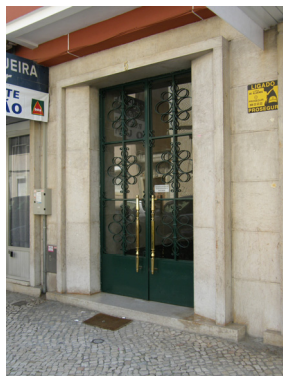
Door of the building
