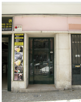
Door of the building
