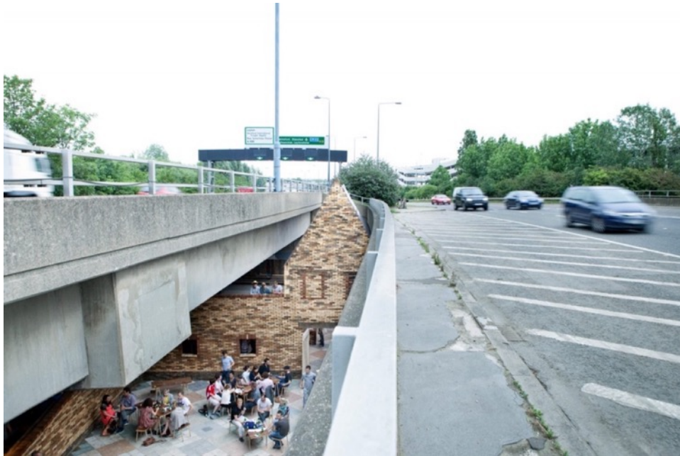
Figura 138. "Folly for a Flyover", Assemble, 2011. Foto: ©David Vintiner. Fonte: Assemble website. https://assemblestudio.co.uk/projects/folly-for-a-flyover
