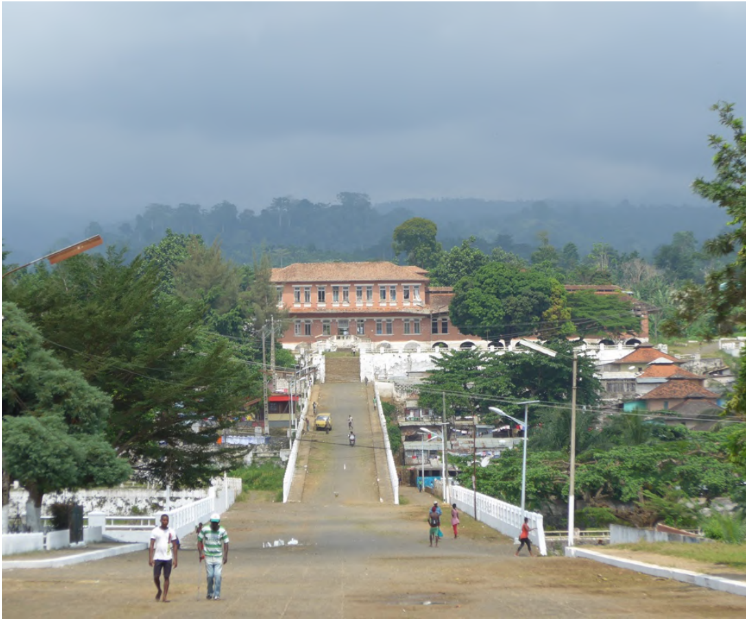
Fig. 2. Roça Augustinho Neto (Rio do Ouro), view from the location of the main plantation house towards the massive hospital building in 2015 (Photograph: author).
