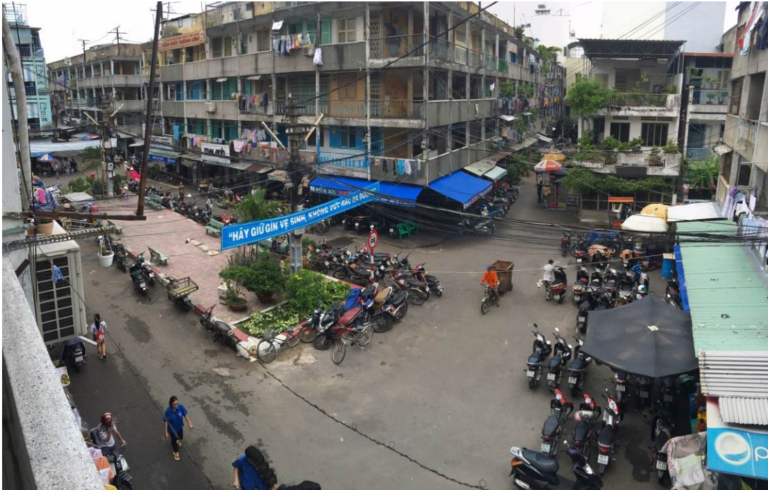
Figure 4. Public Park in front of Block D. On the top right, rows of residential house were built at the heart of the CC's area (Photographed by Loc Tran, 2016)
