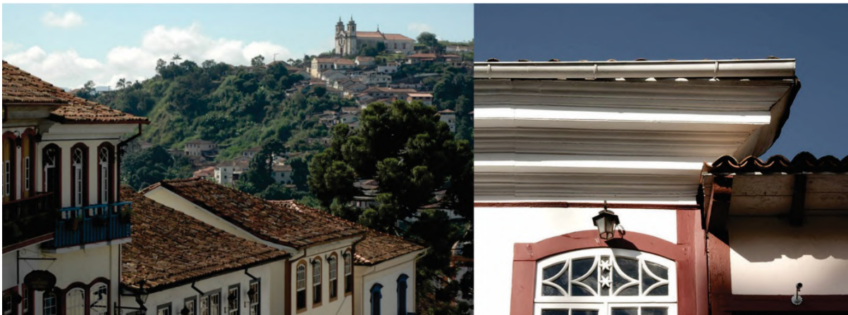
Fig.1. Ouro Preto's landscape and eaves details (IPHAN, 2018).
