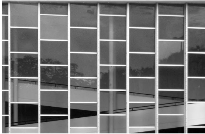
3. View of the circulation ramps, Miguel Bombarda Hospital, Maputo, Mozambique, 2012 EWV, Ana Tostões, 2012 ( http://ewv.tecnico.ulisboa.pt )
