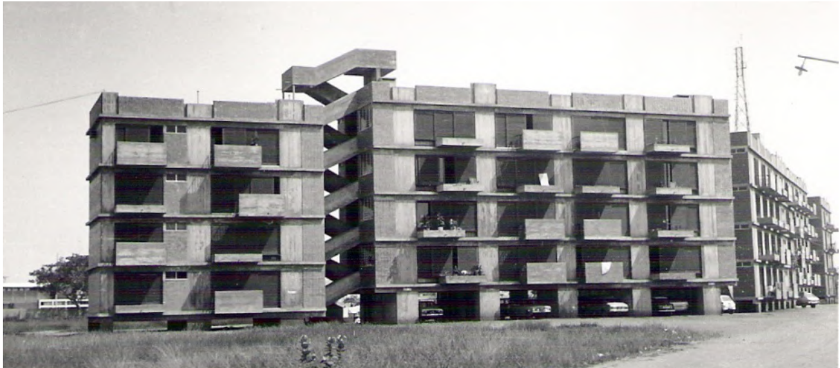
Fig.3. Collective Housing Block built. CTT Neighbourhood, Fernão Simões de Carvalho, Luanda, 1968 (Archive:FSC)
