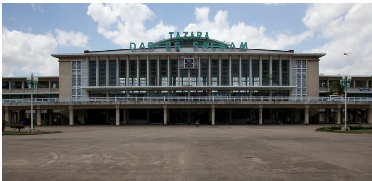
Fig.3. Façade of TAZARA Terminus, Dar es Salaam, Tanzania, 1976. (Source: "TAZARA Railway." Retrieved May 17, 2017, from https://en.wikipedia.org/wiki/TAZARA_Railway .)
