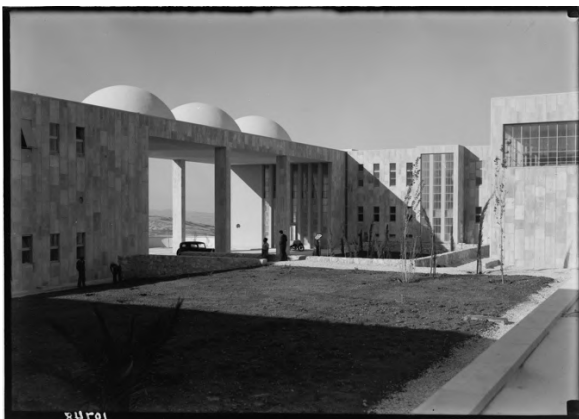
Fig.14. Hadassah Hospital, Detail, entryway domes.
