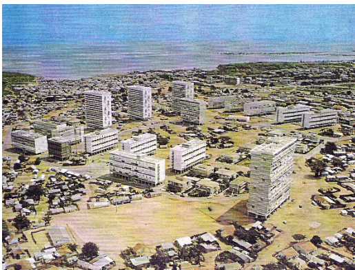
Fig.9. Prenda under construction (1960 decade). Source: Simões de Carvalho archive.
