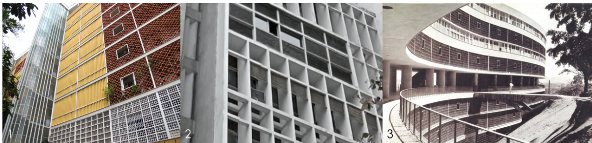
Figure 1: Guinle Park, Lúcio Costa, 1953. Brises and different formats of Cobogos used in the closing of the volume. Fig.2: Brothers MMM Roberto, Housing Building, 1945. These architects made different uses of the sunshades as aesthetic for the building. Fig 3.: Pedregulho Housing Set, Affonso Eduardo Reidy, 1943. Social housing building, of the few that makes use of a curvilinear plant to suit the land and uses the raw ceramic bricks to close the building and ensure natural ventilation.
