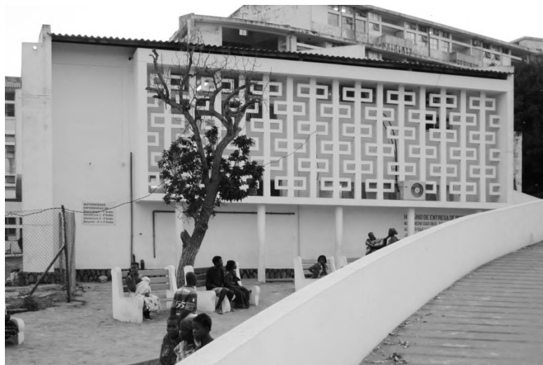
10. Exterior view, façade details, Nampula, Mozambique, 2010 EWV, Ana Tostões, 2010 ( http://ewv.tecnico.ulisboa.pt )
