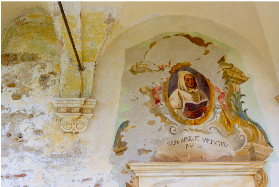
Fig. 8 – Painting on the top of “O” cell in the north arm. Decay phenomena show the different paint layers (white, yellow, green), the plaster cut surrounding the painting and traces of green paint close to the painting (photo by the authors, March 2019).
