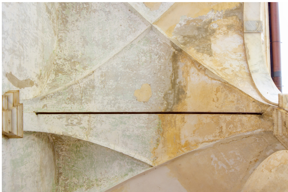
Fig. 3 – Vault intrados in the south arm. Green paint traces are appearing under two layers of different yellow paint (photo by the authors, March 2019).
