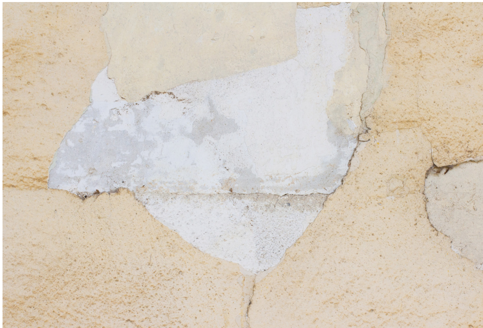
Fig. 9 – Horizontal plaster cut on the south arm and two different yellow paint layers (photo by the authors, October 2019).
