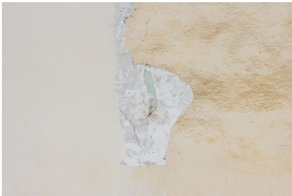
Fig. 5 – Two different plasters between the sixth and seventh spans of east arm. The colour, the thickness and the grain are clearly different (photo by the authors, October 2019).
