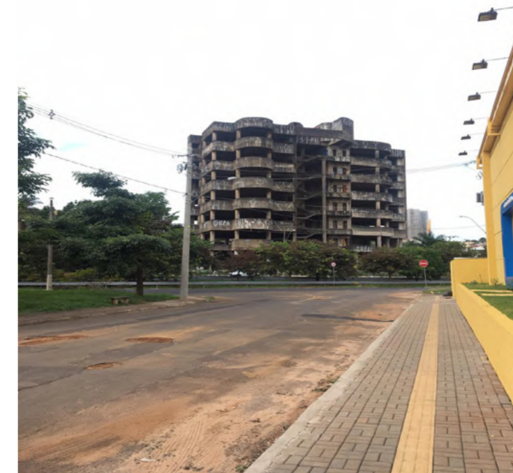
Figure 2 – Abandoned building in study. Source: Personal Archive (2019).
