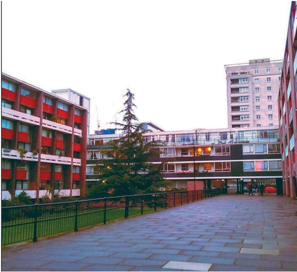
Figure 2. Chamberlin Powell & Bon—Basterfield House and Stanley Cohen House, Golden Lane Estate, Central London (1952–1962)—photograph by João Cunha Borges.
