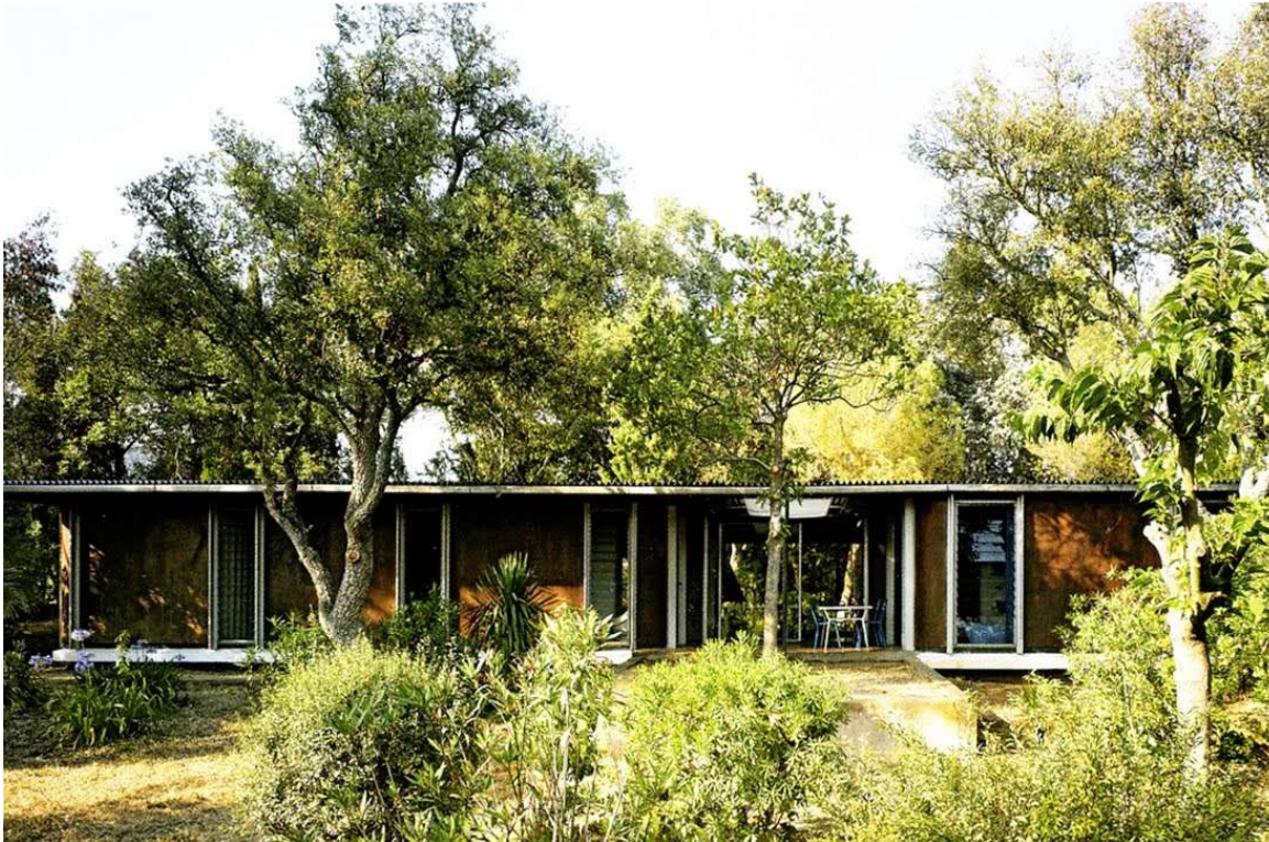
Maison Seynave. (Fonte: http://www.diedrica.com/2014/09/seynave-vacation-house.html )..
