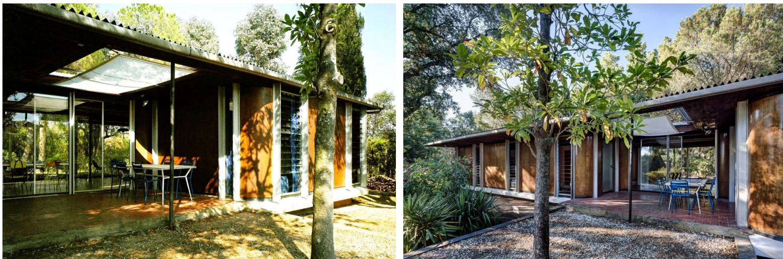
Maison Seynave. (Fonte: http://www.diedrica.com/2014/09/seynave-vacation-house.html ).
