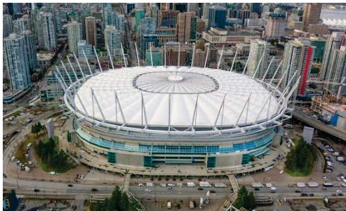
Figure 7. BC Place Stadium – roof closed
