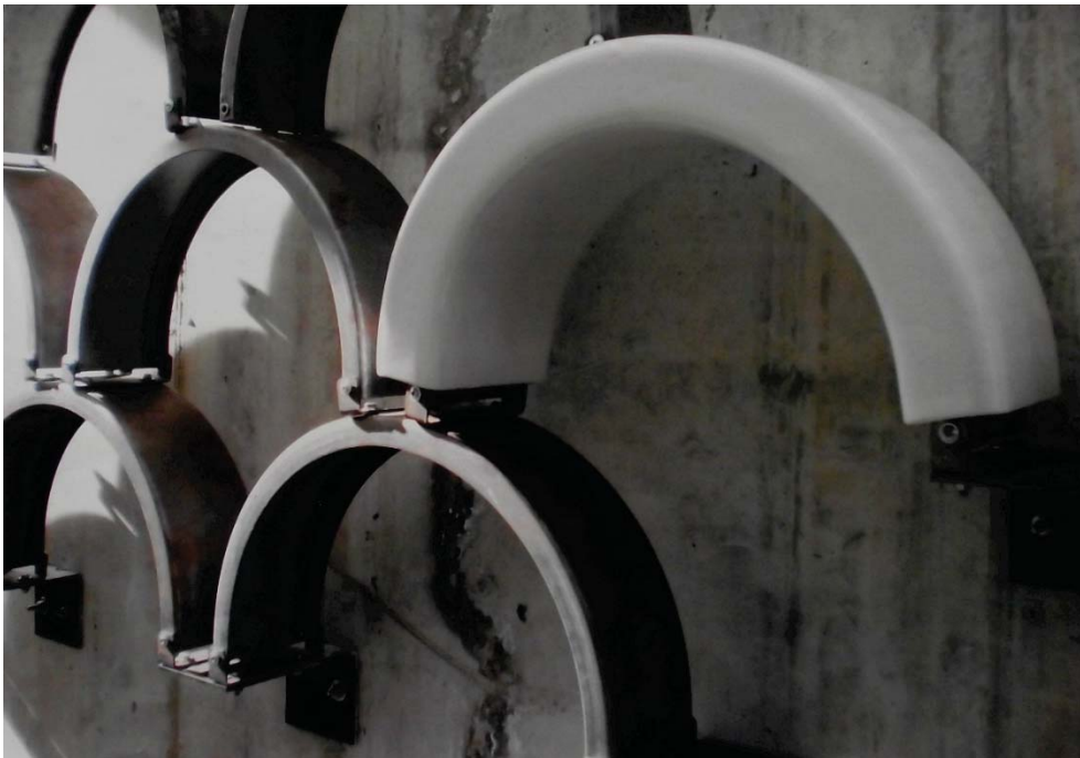
Figure 6. Lisbon Aquarium construction of the façade, Lisboa, Portugal. (Photography by Campos Costa Architects).
