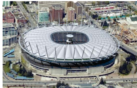
Figure 8. BC Place Stadium – roof open
