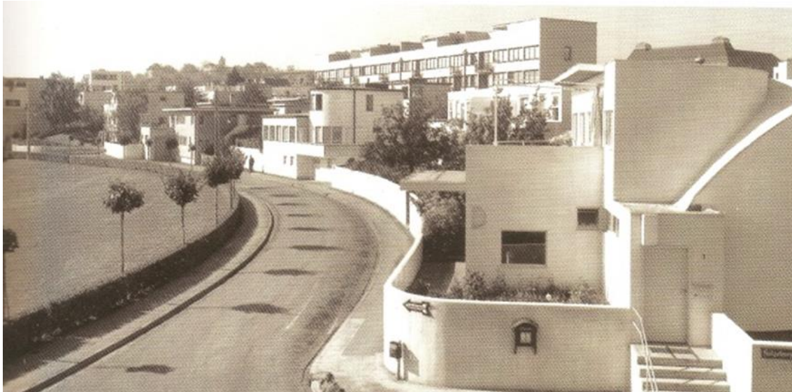
Fig. 3. Vista geral de Weissenhof de Stuttgart, 1927. Em, JONES, Peter Blundell, Modern Architecture Through Case Studies . Woburn MA: Architectural Press, 2002, p.11
