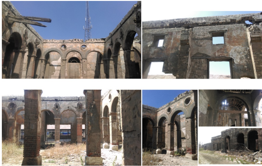
Figure 5. Shows the site of study and its existed condition (9)
