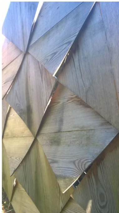
Figure 1. Ray 2 – Prototype after Three Years of Being Exposed to Weather (photo: Davidová 2016)
