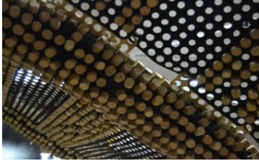
Figure 10 – Cork used as a membrane
