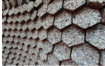
Figure 11 – Cork used as a finishing material
